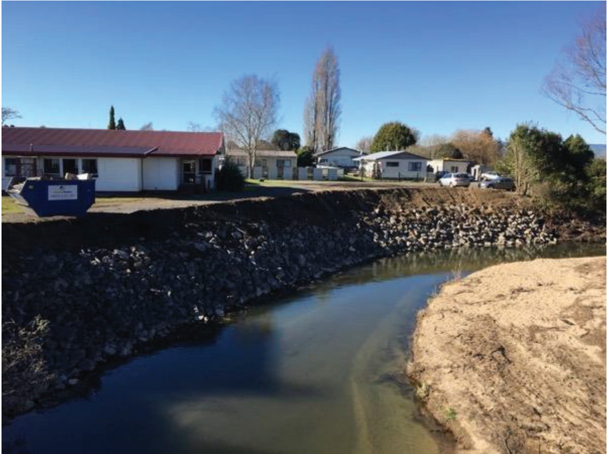
Figure 19: Rock revetment works and vegetation removal Parawai Marae (Post event)
