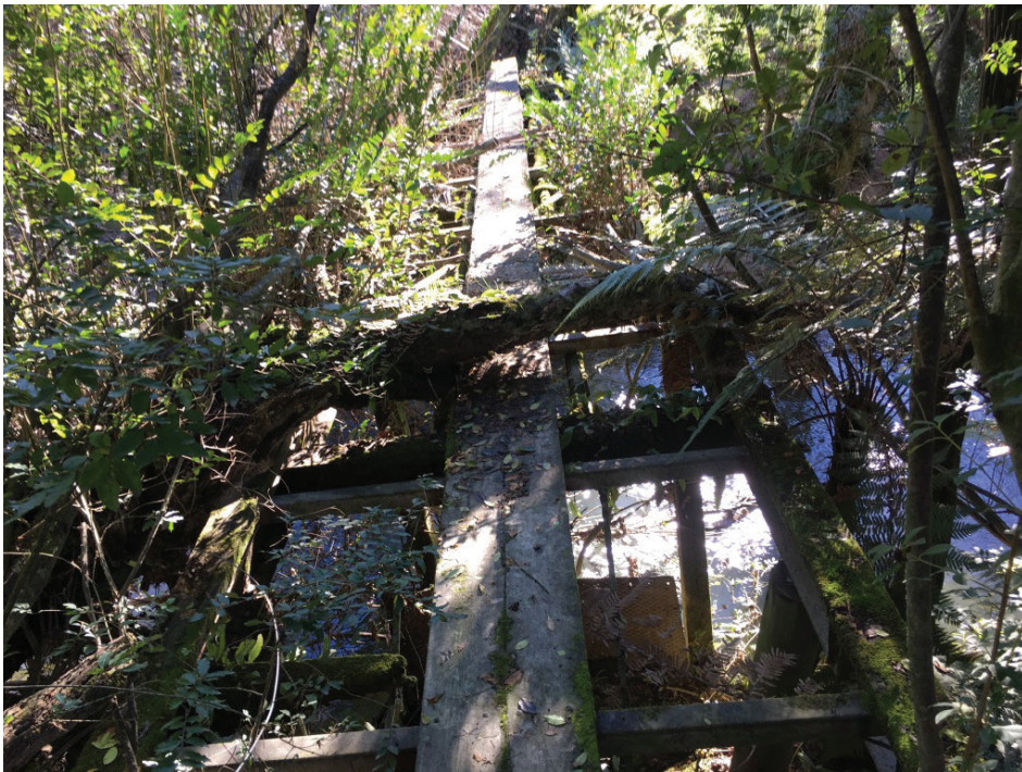
Figure 26: Notable Channel Obstructions Ngongotahā Stream (Agrodome Property)
