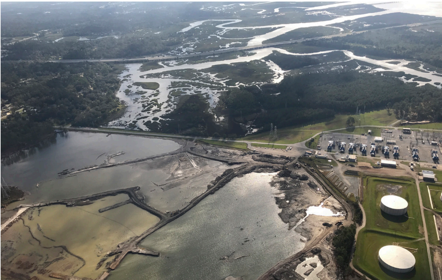
At Plant McManus, unknown amounts of coal ash spilled into Georgia's Golden Isles during Hurricane Irma in 2017. (Courtesy of Jen Hilburn / Altamaha Riverkeeper)
