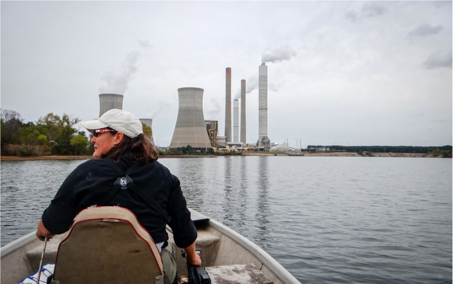
Altamaha Riverkeeper Jen Hilburn near Plant Scherer. The groundwater at Plant Scherer is unsafe, particularly around the ash pond. (Courtesy of Jen Hilburn / Altamaha Riverkeeper)
