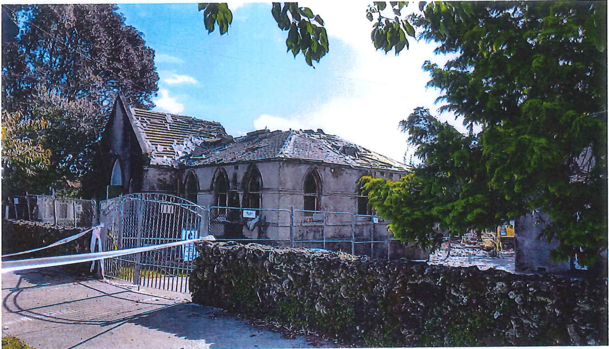
Photograph 1: Vestibule and front northern annex facing Esplanade Road.
