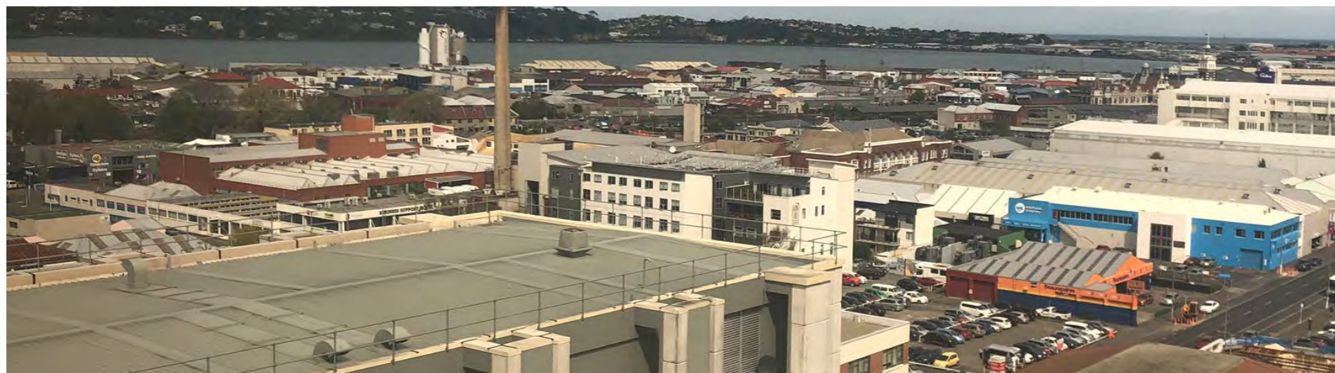
Figure 17. View Over-looking the new hospital site and harbour basin.
