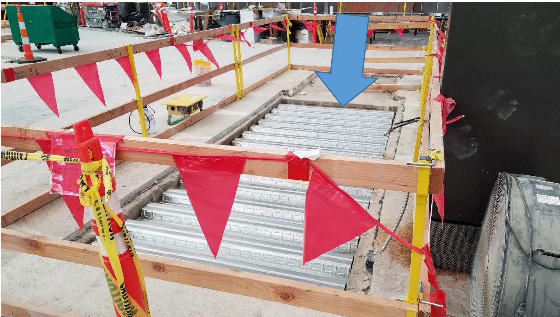
L5 plaza, north bridge escalator pit infill. (12/13/18)
