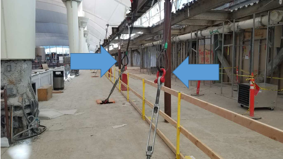
L6 clerestory cable relocation tie-ins hung. (Looking north, 12/19/18)
