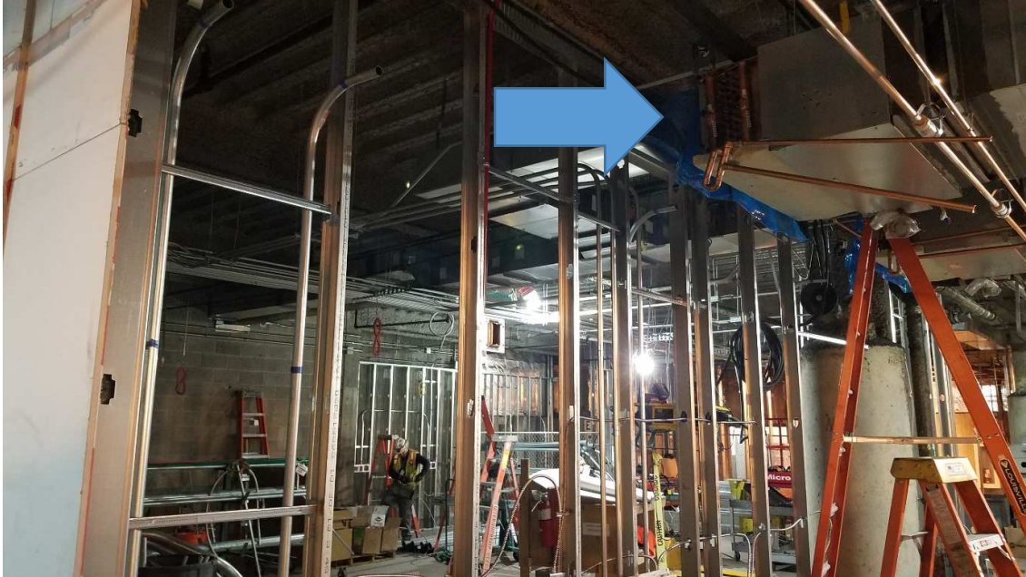
CMF framing and overhead MEP installation. (12/19/18)
