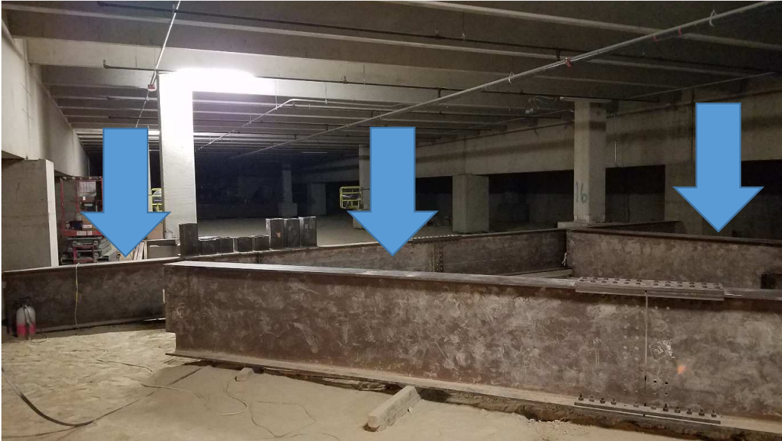
L3 Crawl space with steel for escalator pits. (12/19/18)
