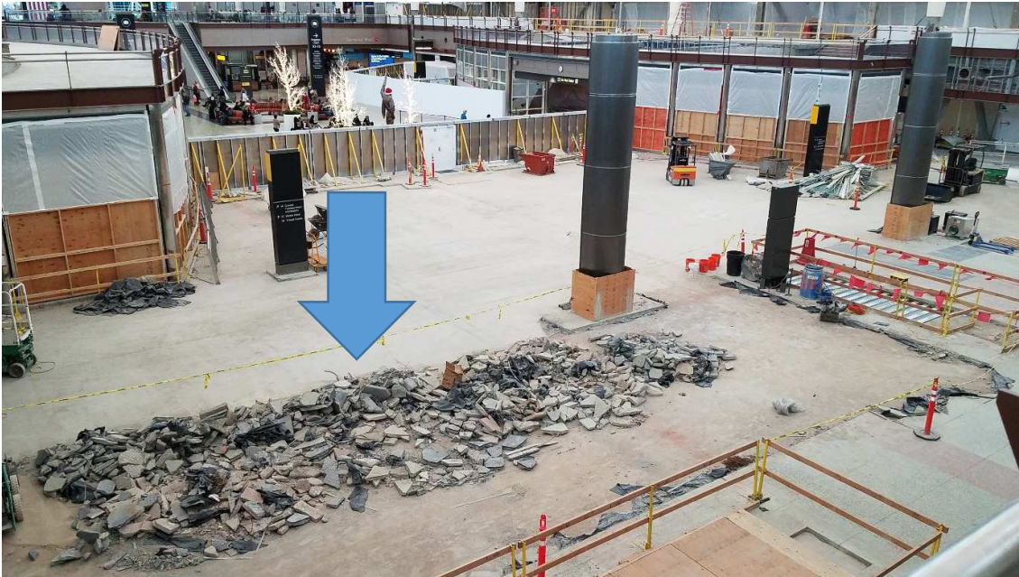
Plaza flooring demolition and AGTS glass removal. (Looking south, 12/19/18)
