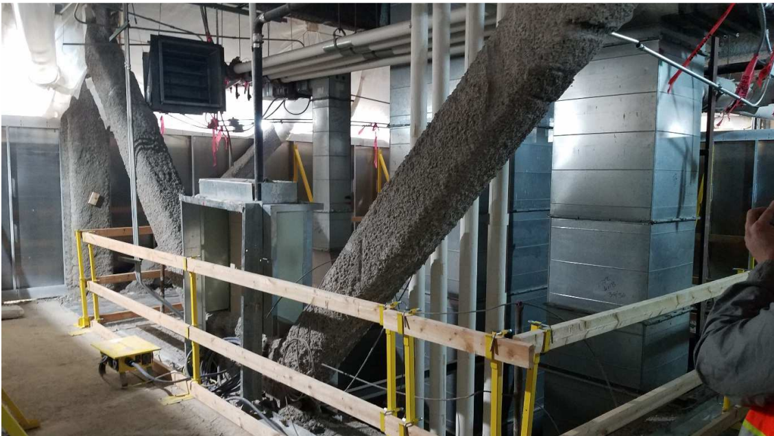
L6 west mechanical shaft architectural demolition. (12/19/18)
