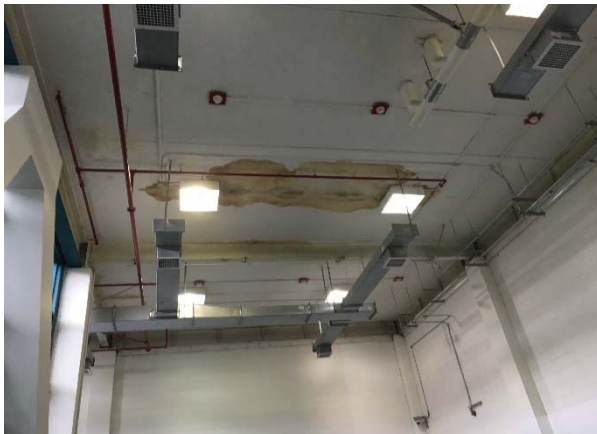
Figure 4. Roof leaks found in every housing unit.
