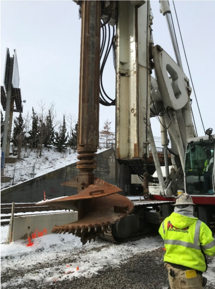
Viaduct Drilled Shafts
