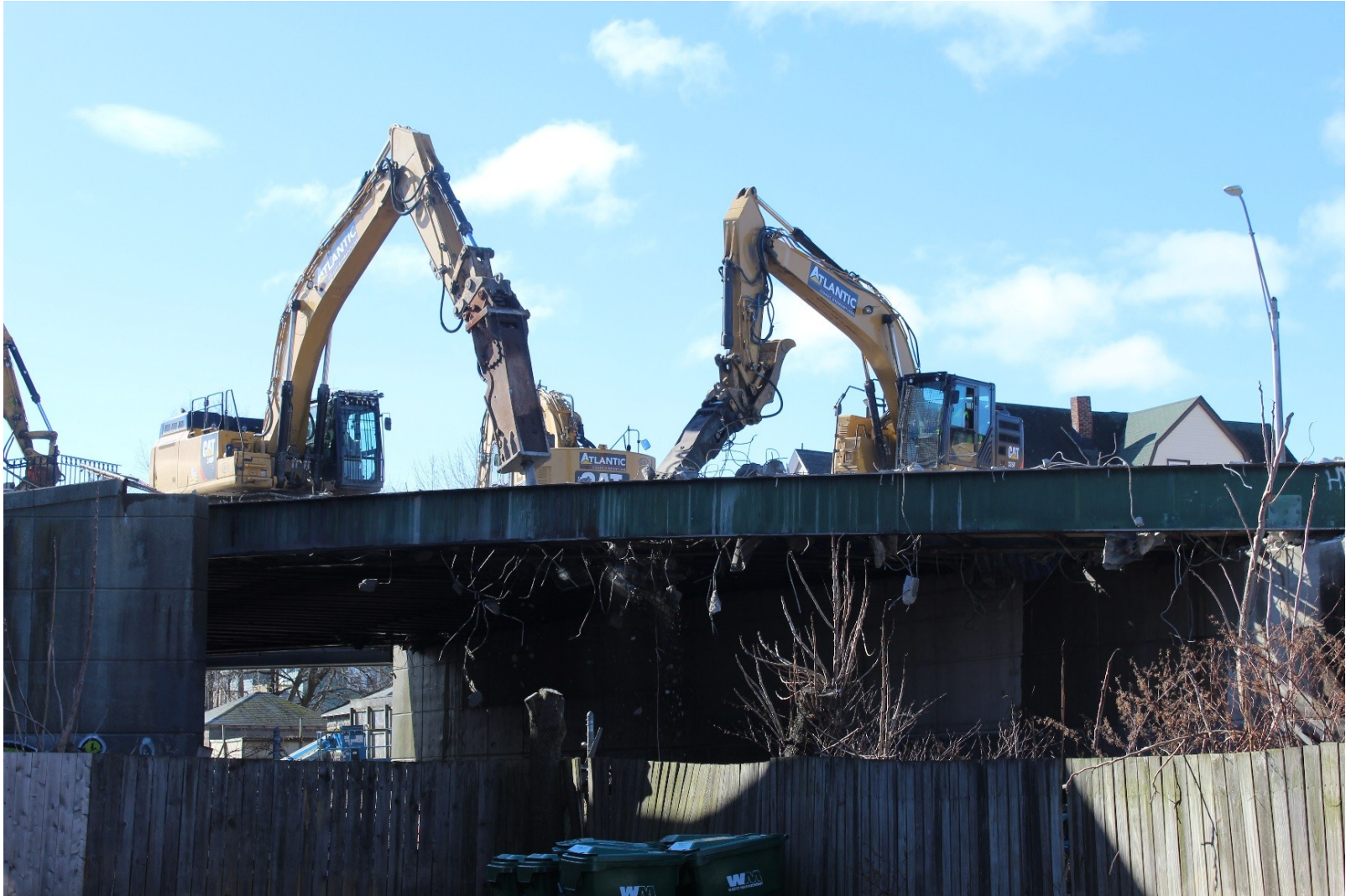
Broadway Bridge deck demolition
