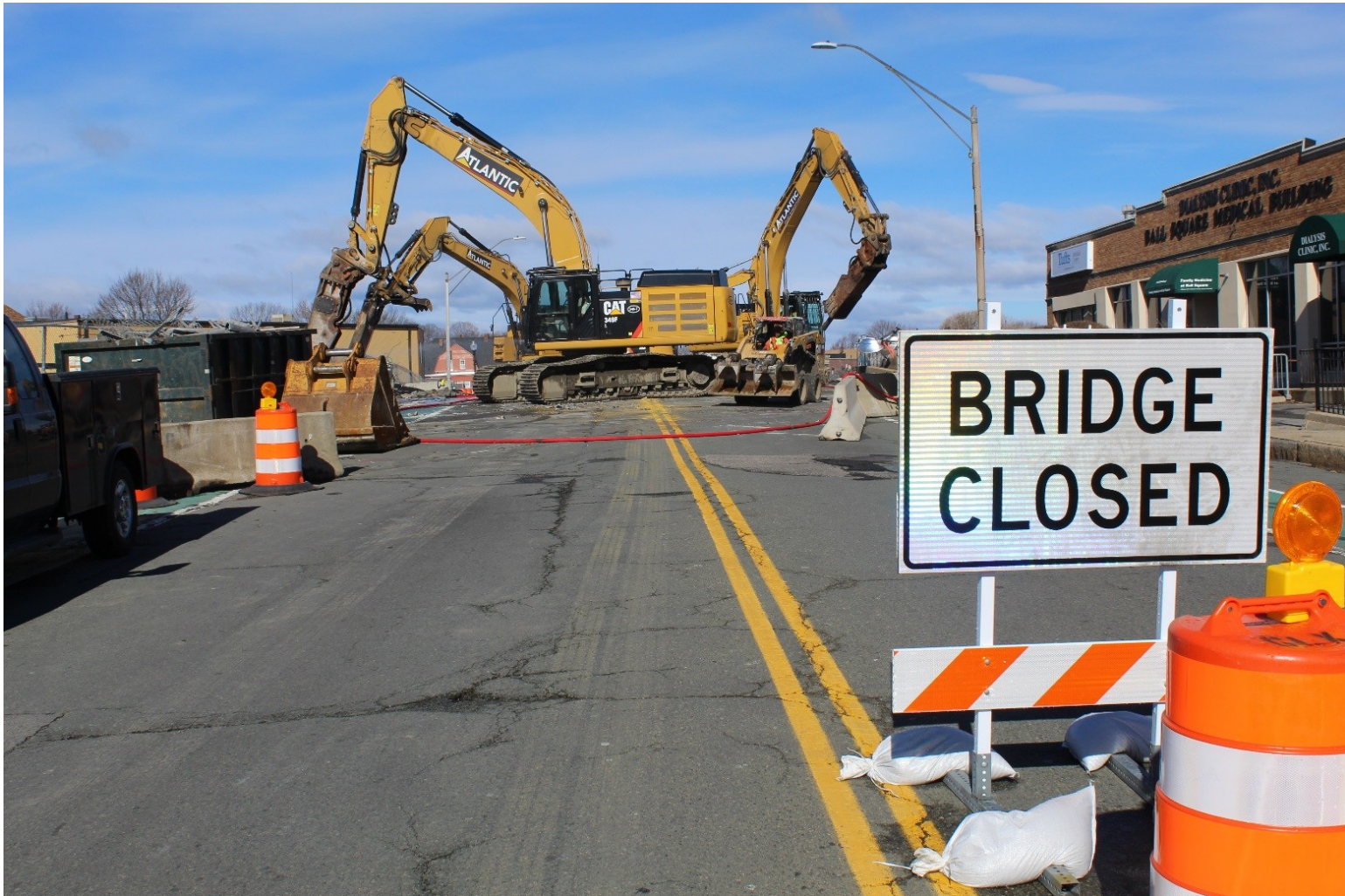
Broadway Bridge deck demolition
