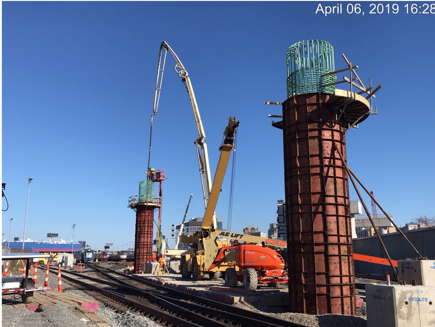
Viaduct Column Installation
