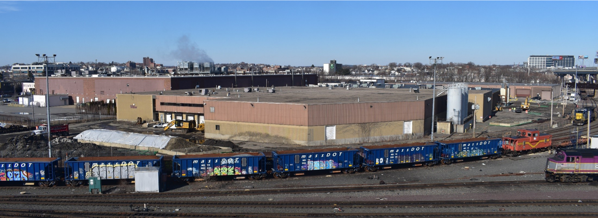
Future Vehicle Maintenance Facility (before building demolition)
