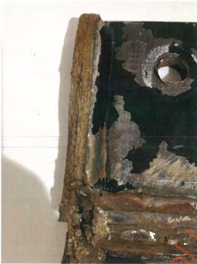
Figure 19 Plate rupture markings, stage III
