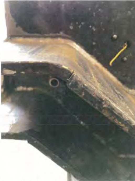
Figure 28 Cut-out in top stiffener, close-up.
