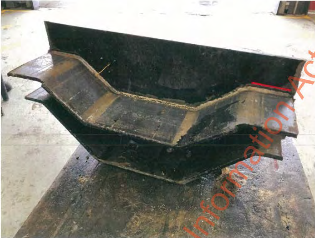
Figure 5 Drawbeam front section rear view, cracks below red line
