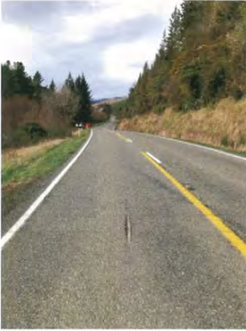
Figure 23 Road section where accident occurred
