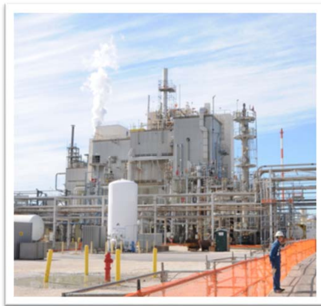
Figure 1. The Lannate ® Manufacturing Building. The methyl mercaptan release occurred in the manufacturing building. Source: CSB.
