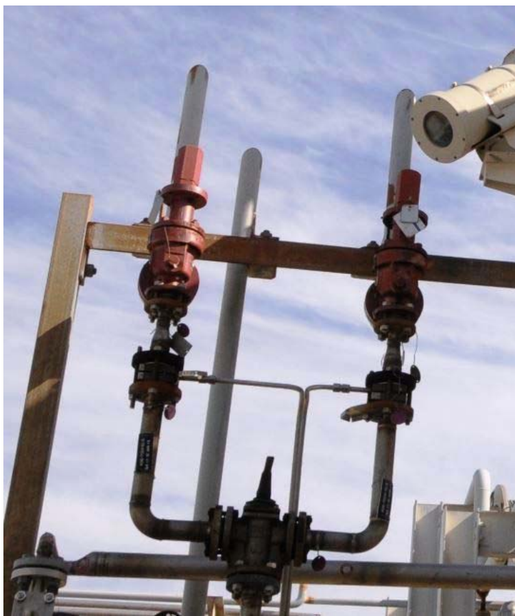
Figure 33. Nitrogen Relief Valves at One of the Two Methyl Mercaptan Railcar Unloading Stations. DuPont PHAs and relief valve design documents never considered the possibility of lining up the methyl mercaptan storage tank pumps to these relief valves—as they were at the time of the incident. As a result, liquid methyl mercaptan was discharged from a system designed for nitrogen vapor. Source: CSB.
