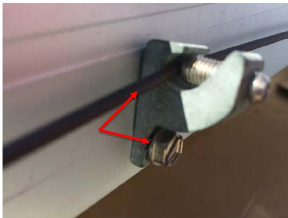
Image of Improper Module Grounding (Washer Should be Between Lug and Module Frame)
