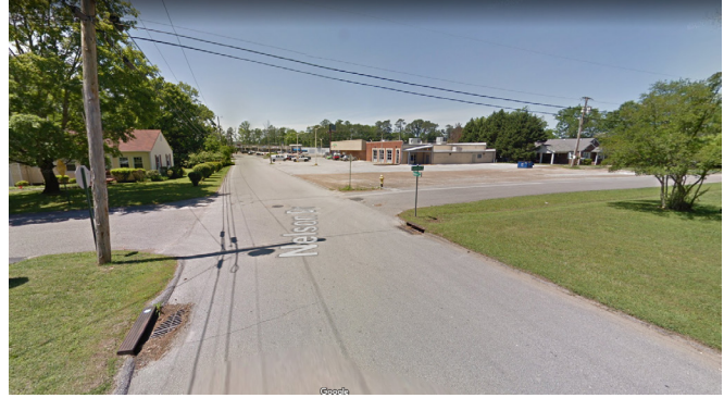
NELSON DRIVE, A FEEDER ROAD CONNECTING A RESIDENTIAL NEIGHBORHOOD TO A COMMERCIAL NODE ON LEE HIGHWAY LACKS BASIC INFRASTRUCTURE INCLUDING SIDEWALKS, CURBING, DRAINAGE AND LIGHTING.
