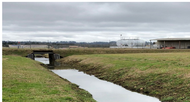
LARGE STORMWATER CONVEYANCE ON AIRPORT ROAD
