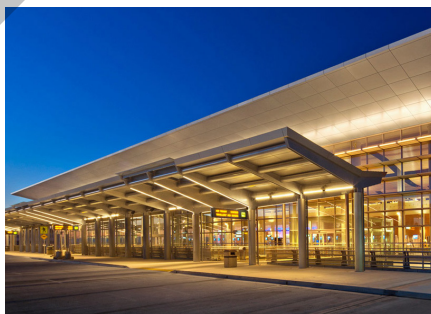
▶ WINNIPEG JAMES ARMSTRONG RICHARDSON INTERNATIONAL AIRPORT
