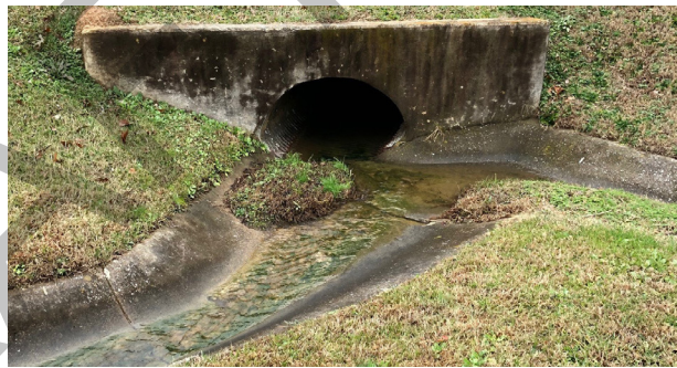
STORMWATER POI #5 ON SHEPHERD ROAD
