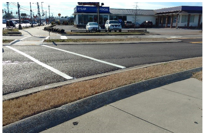
SOME SIDEWALK IMPROVEMENTS HAVE BEEN MADE, BUT THERE IS LIMITED ADA ACCESSIBILITY AND INCONSISTENCIES FROM BLOCK TO BLOCK. THIS IS THE INTERSECTION OF EAST BRAINERD. ROAD AND LEE HIGHWAY.
