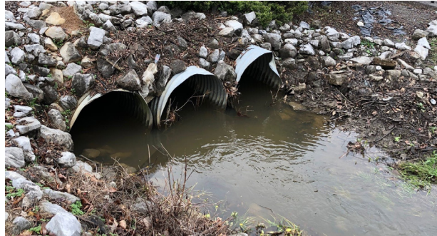
STORMWATER POI #12 ON AIRPORT ROAD
