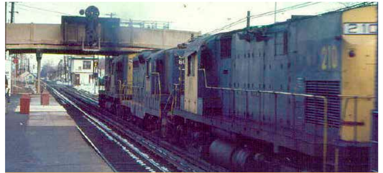
Afternoon freight RF-60 heads east under the Mineola Blvd. Bridge, ahead of the rush hour. March 1, 1977. The bridge has been rebuilt with higher clearances that could allow for larger freight trains to pass, notes Jack Martins, a former Mineola mayor and later state senator who was a vocal opponent of the 2005 third track plans. © Tim Darnell, RRPictureArchives.net
