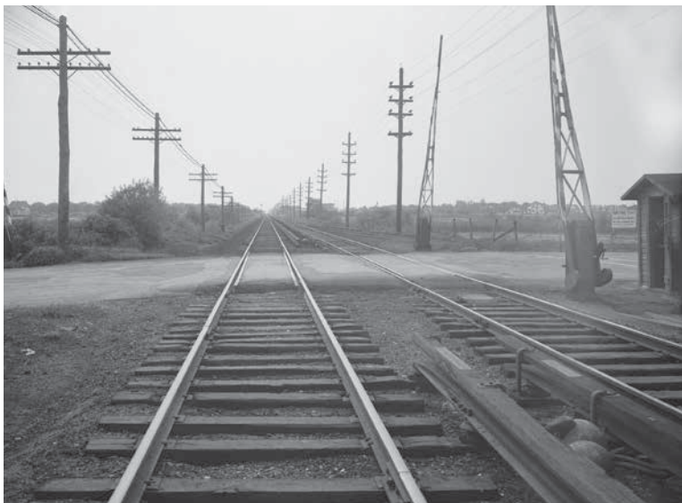
Mineola’s deadly Herricks Road crossing in 1939, two years before its first major accident. On the right is the hut for watchmen tasked with lowering the gates. In the pasture behind it is a sign offering 7 acres zoned commercial/industrial. © Estate of Frederick J. Weber. Courtesy of the Queens Borough Public Library Archives, Frederick J. Weber Photographs
