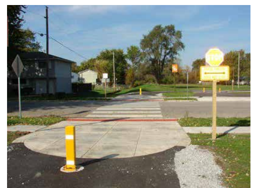
Example of Concrete Node with Bollard
