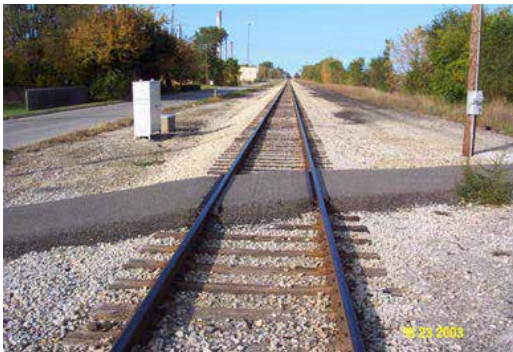
Rubber Panel Rail Crossing - Amtrak Rail Line Michigan City, IN
