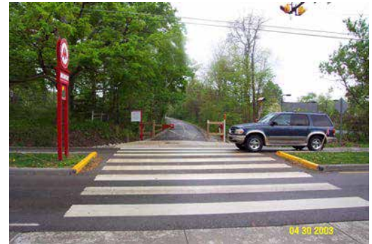
Shared Use Trail Street Crossing Monon Trail - Carmel, IN
