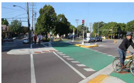
EPOXY COATING ON ASPHALT
