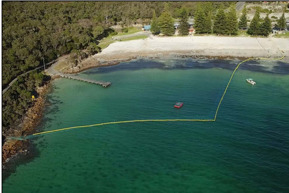
Figure 28. Global Marine Enclosures “semi-rigid” barrier installation, Middleton Beach, WA. Photo credit Google Earth. Retrieved 15 September 2019.
