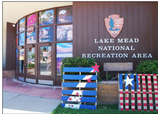
One-way vinyl window film with nature photographs provides security for the front desk attendant at a National Park Service field unit.
