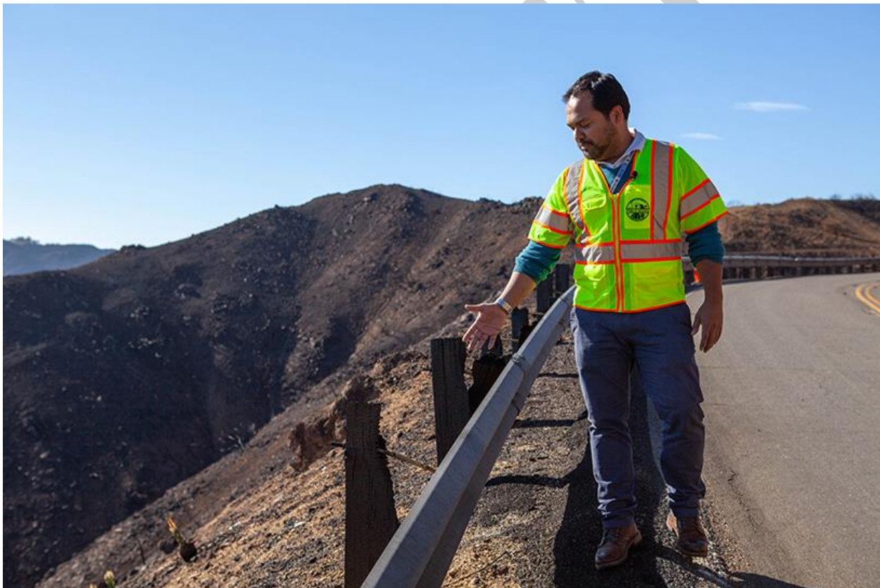
Figure 5—Infrastructure Damage – Canyon Road
