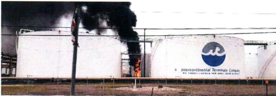
Early Photograph of Fire at Manifold Tank 80-8
