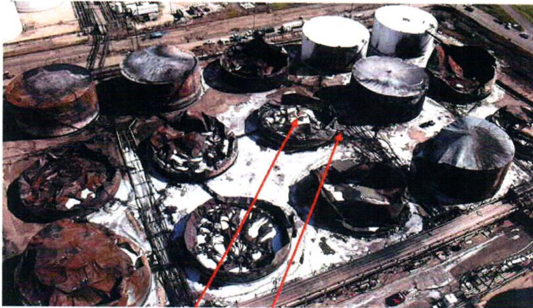
Tank 80-8 and Manifold, Origin of Fire
