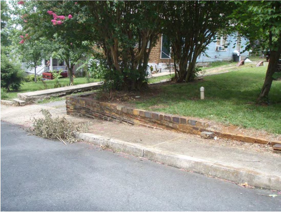
Stop 8a - Wall at Falls Road and Stanly Street Made of Furnace Brick
