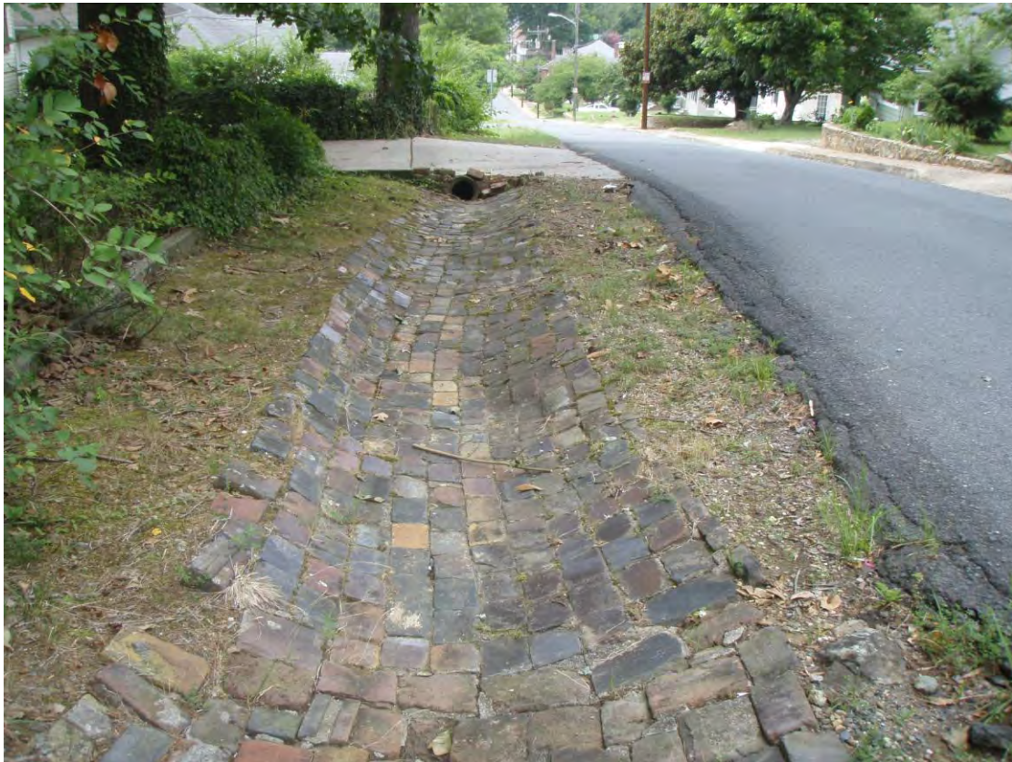
Stop 8a - Storm Drain at Falls Road and Stanly Street Made from Furnace Brick
