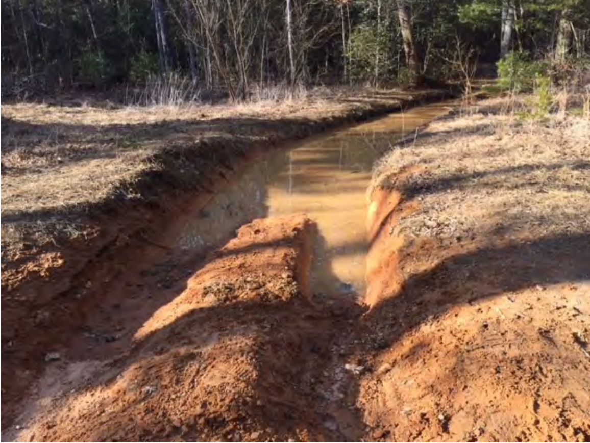
Photo 11 Forest Road Damage that is Impacting Soil and Water Resources and Visitor Safety and Enjoyment
