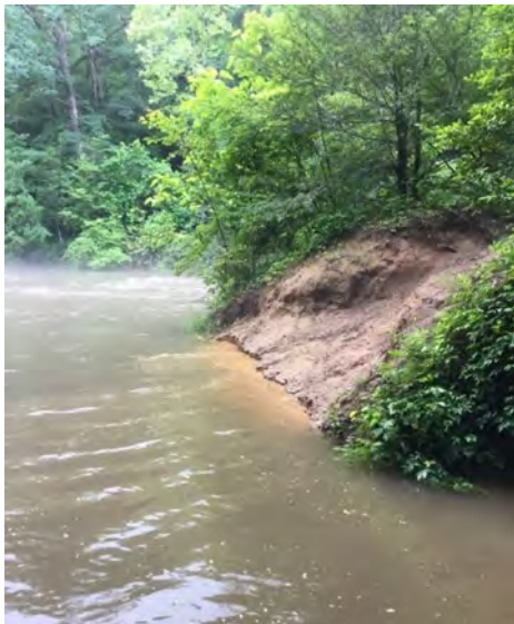
Photo 3 Streambank Erosion Cause Increased Sedimentation, Negatively Affecting Water Quality and Aquatic Wildlife Habitat. Example along Warwoman Creek Shown Here.
