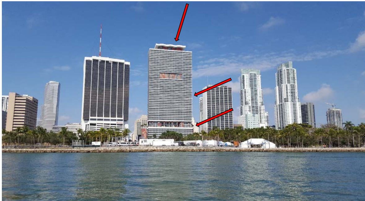
Figure 1 - 2. View of 50 Biscayne Condominium building from bay, after festival during removal of Ultra equipment, showing outside test locations.
