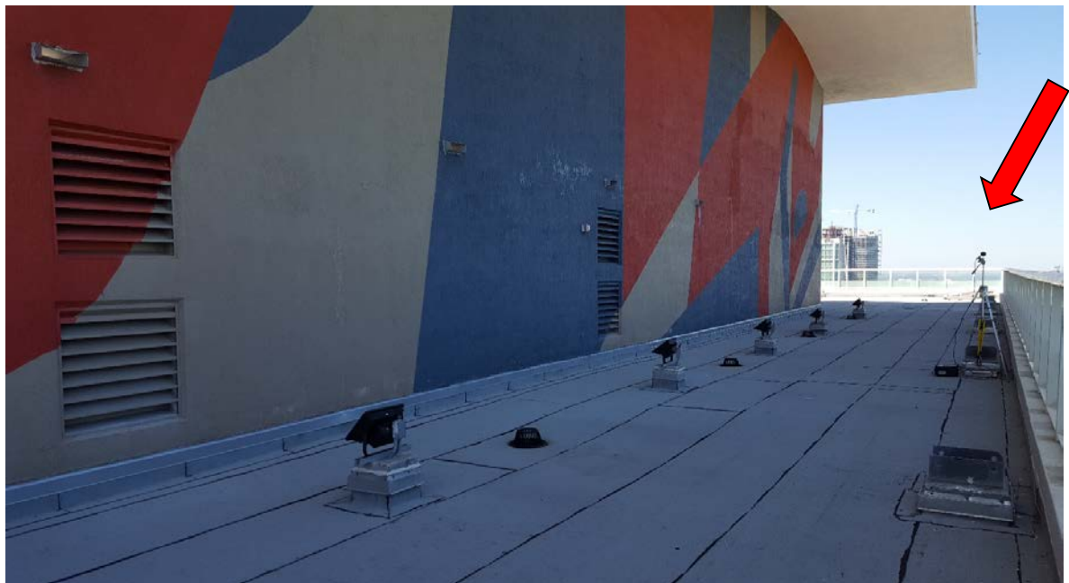
Figure 1, f. Long Term Test Position L2 - building roof.
