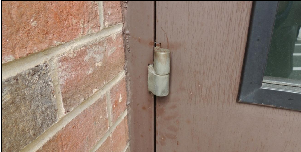
Figure 18: Exterior door with protective hinge covering.
