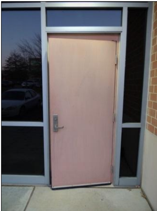
Figure 155: Unprotected hinges.
