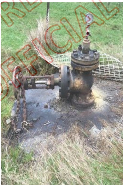
Figure 31 – Blackwater-1 Well (prior to cage being installed)
