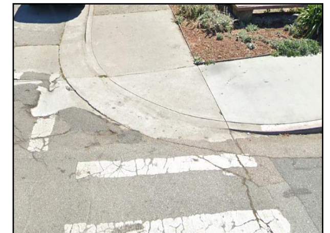
Civil Figure 6: Curb ramp on Locust & Center Street
