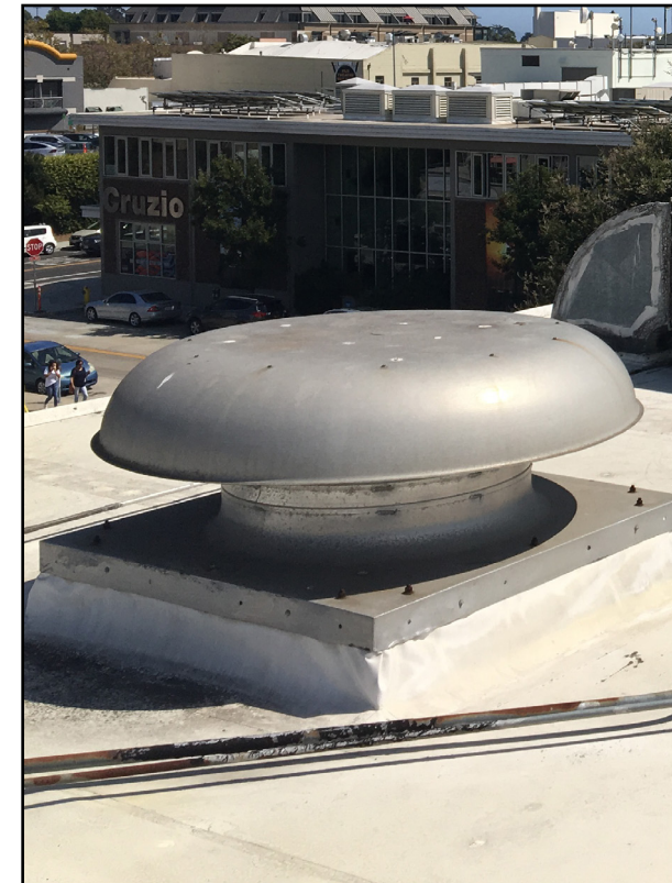
Mechanical Figure 9: Building Relief Hood
