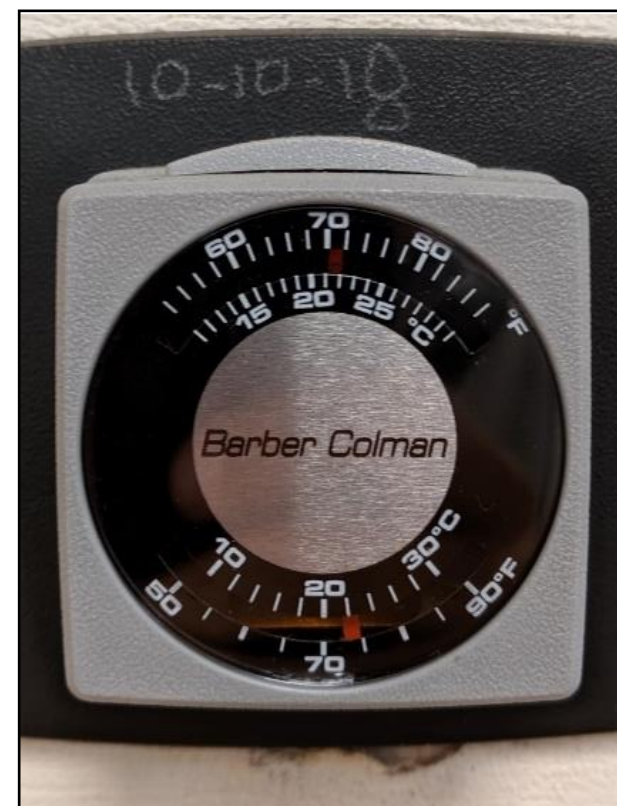
Mechanical Figure 15: Pneumatic Thermostat
