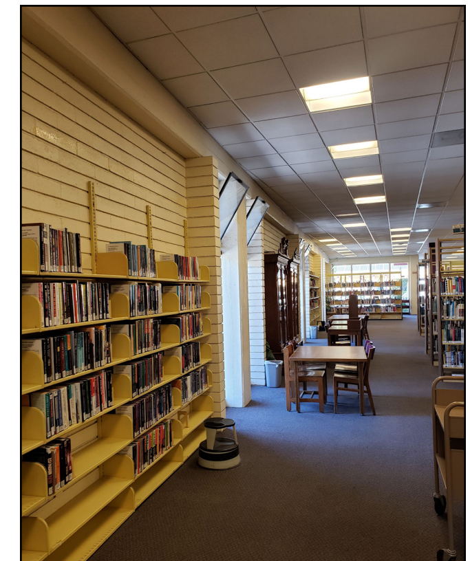
Concrete block walls at 1-story section
