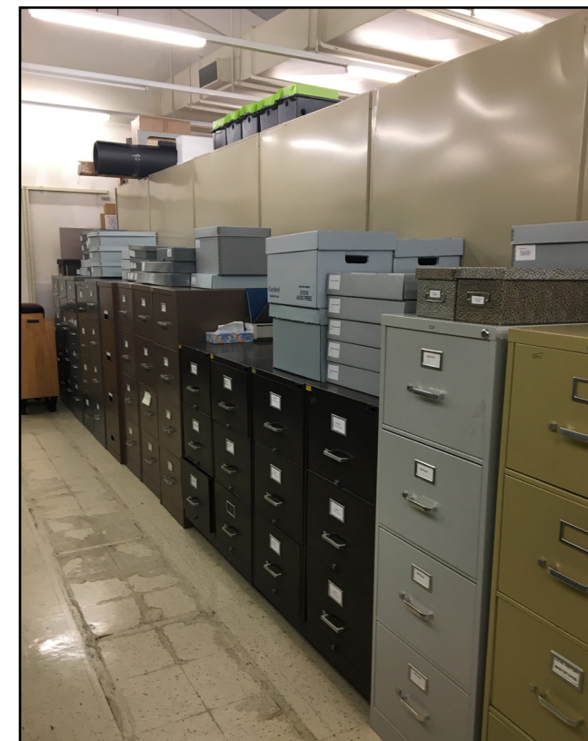
Aging and damaged floor tiles
