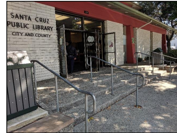
Civil Figure 1: Library main entry on Church Street
