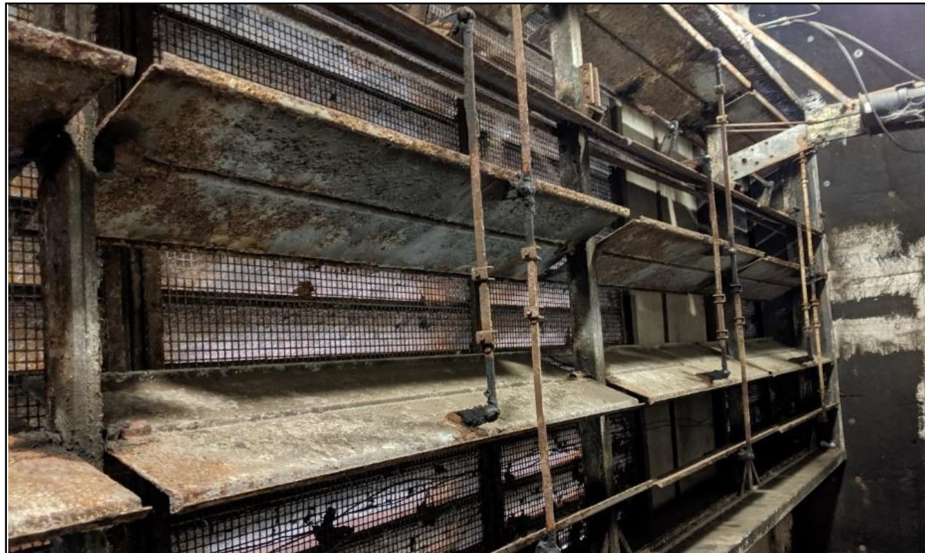
Mechanical Figure 1: AHU Modulating Mixing Dampers
