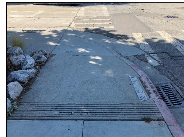
Civil Figure 5: Curb ramp on Church & Center Street
