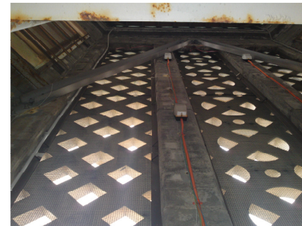
Figure 2: Precast concrete screens in the upper belfry.
