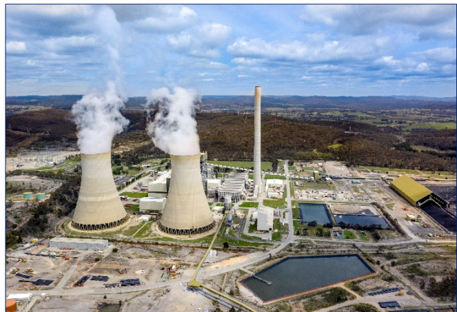
Mount Piper coal power station in Portland, NSW, Australia. Getty Images / mikulas1
