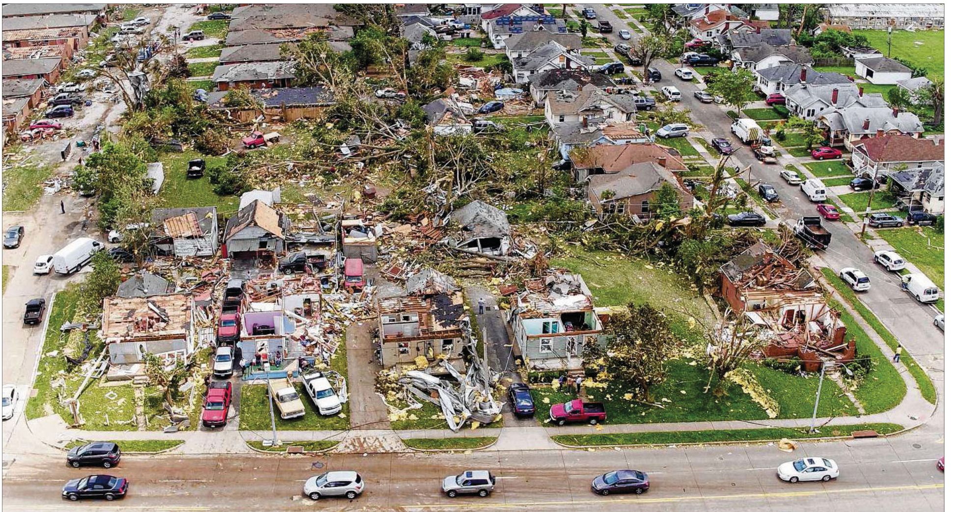
Houses in the Old North Dayton neighborhood along Troy Street where a tornado ripped through industrial buildings across the street and then the neighborhood on Monday night. The Miami Valley has suffered tornadoes in the past, but Monday's storm brought three of them that the National Weather Service labeled an EF-3. TY GREENLEES / STAFF
