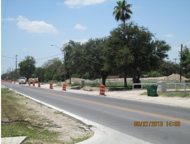
Sam Houston Boulevard Widening
