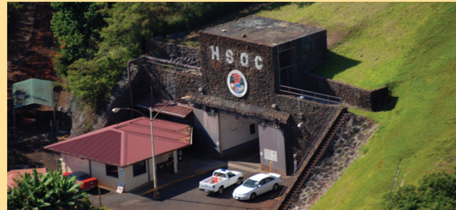
Regional Security Operations Centers, like the one in Hawaii pictured above, provide NSA with the redundancy needed in the event of an emergency.
